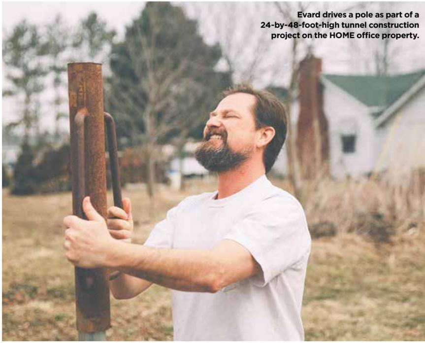
Evard drives a pole as part of a 24-by-48-foot-high tunnel construction project on the HOME office property.
